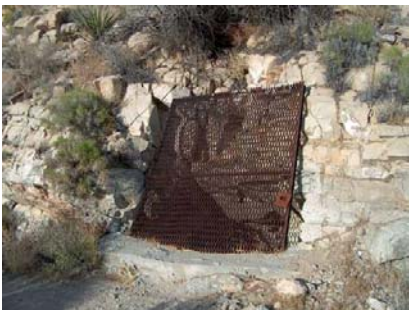
Mine shaft with fencing
